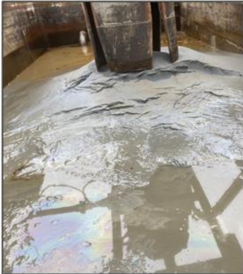
Sand circulated/lifted out of the well
